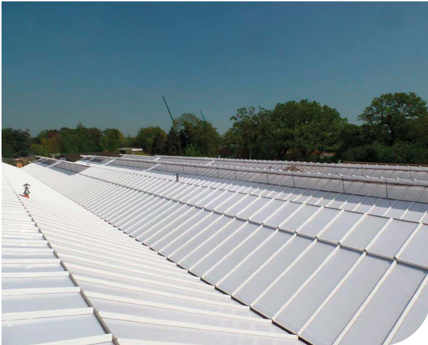
Garden centre project supplied by Areco
